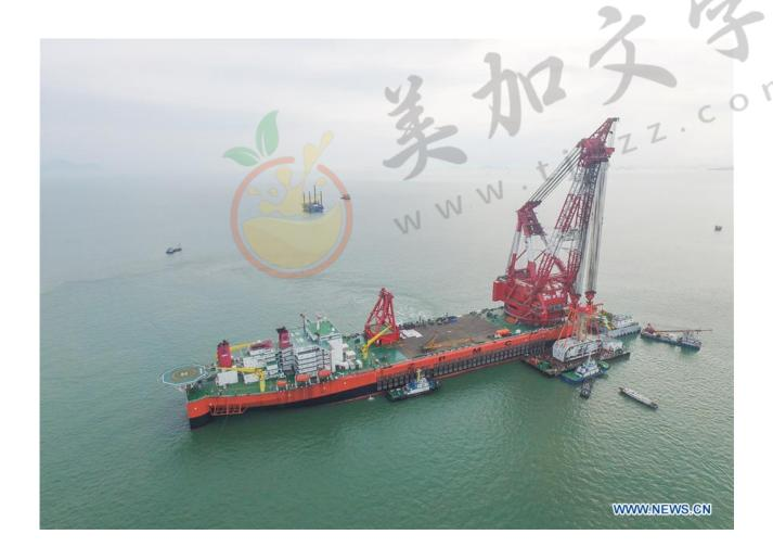
A gigantic crane, which was transformed from a tanker, hoists a 6,000-ton key structure of the world's longest cross-sea bridge linking Hong Kong, Zhuhai and Macao, May 2, 2017. The wedge, 12-meter-long and weighing more than 25 Airbus A380 jets, was lowered to connect the immersed tubes of the underground tunnel of the bridge. The
